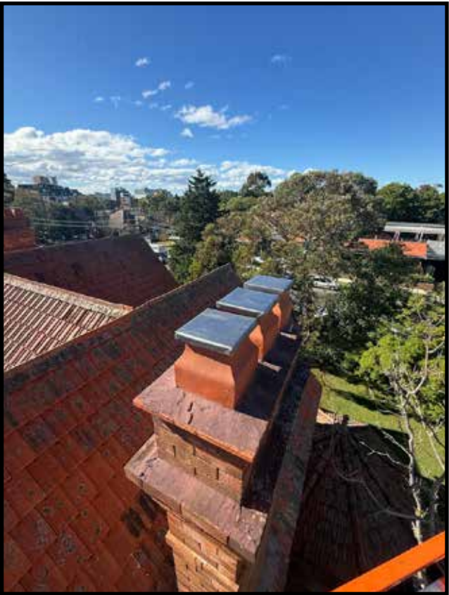
Chimney Capping After
