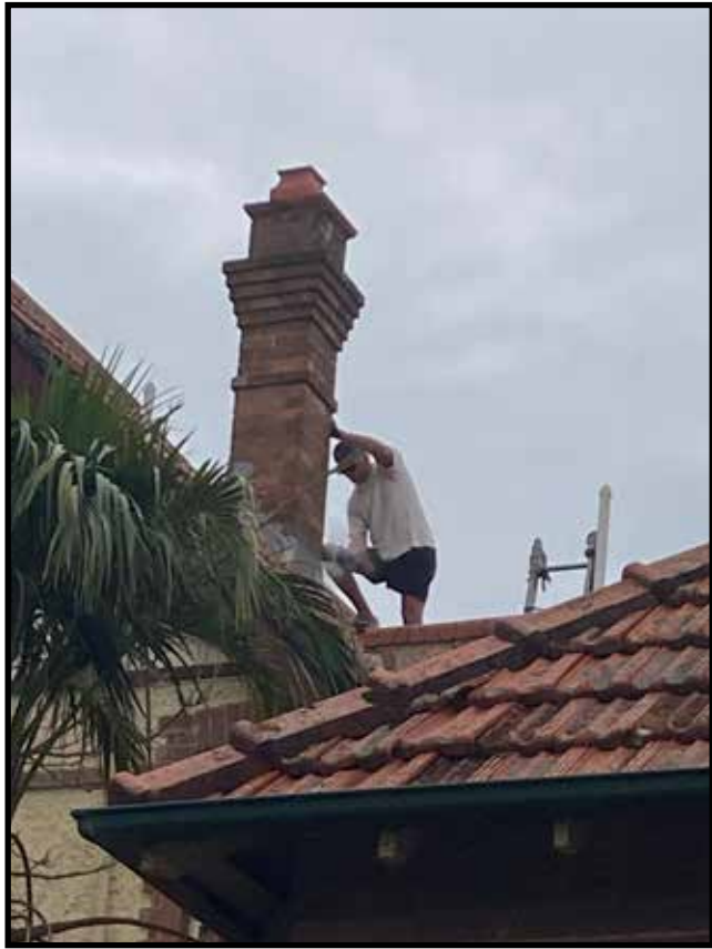
Chimney Works Repairing Lead Flashing
